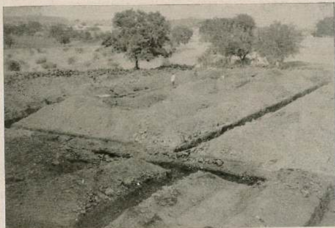
DIGGING THE FOUNDATIONS
