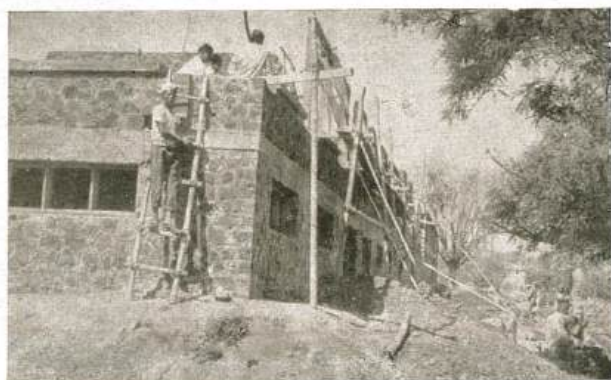
The Corner Basement
