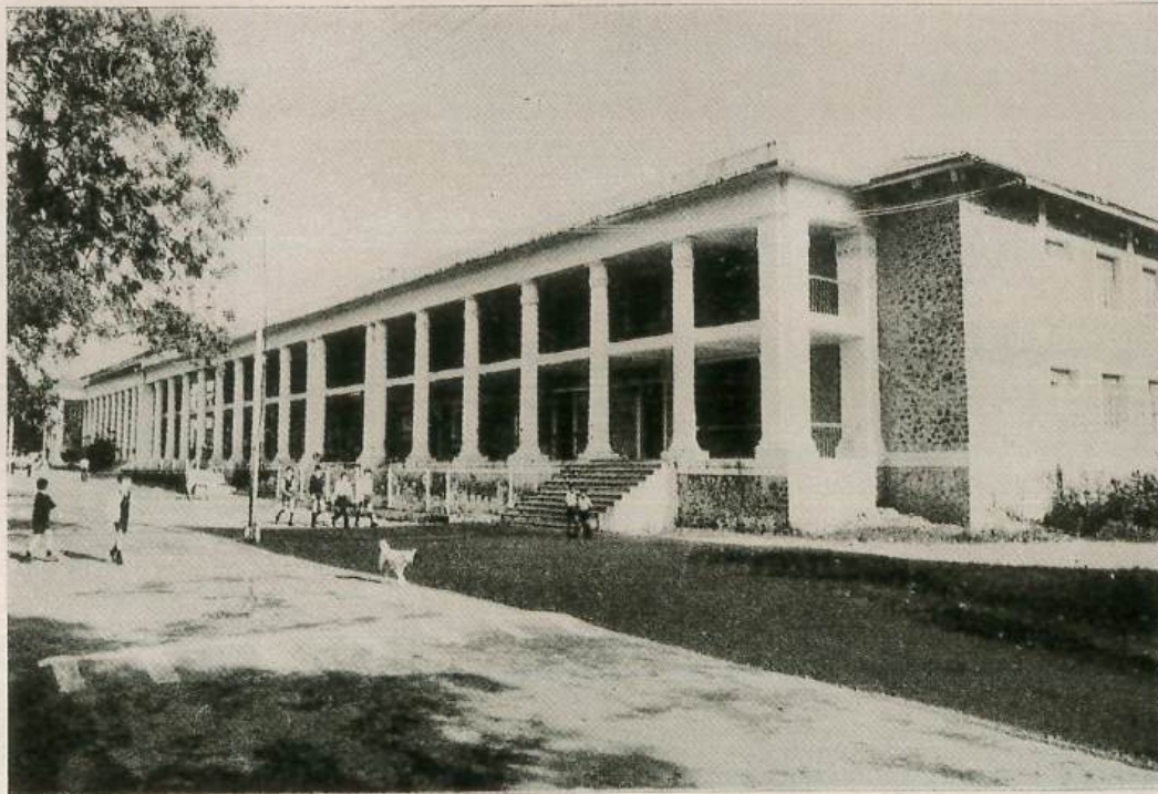
The new addition to Barnes — Junior Academic block with the office and classrooms.
