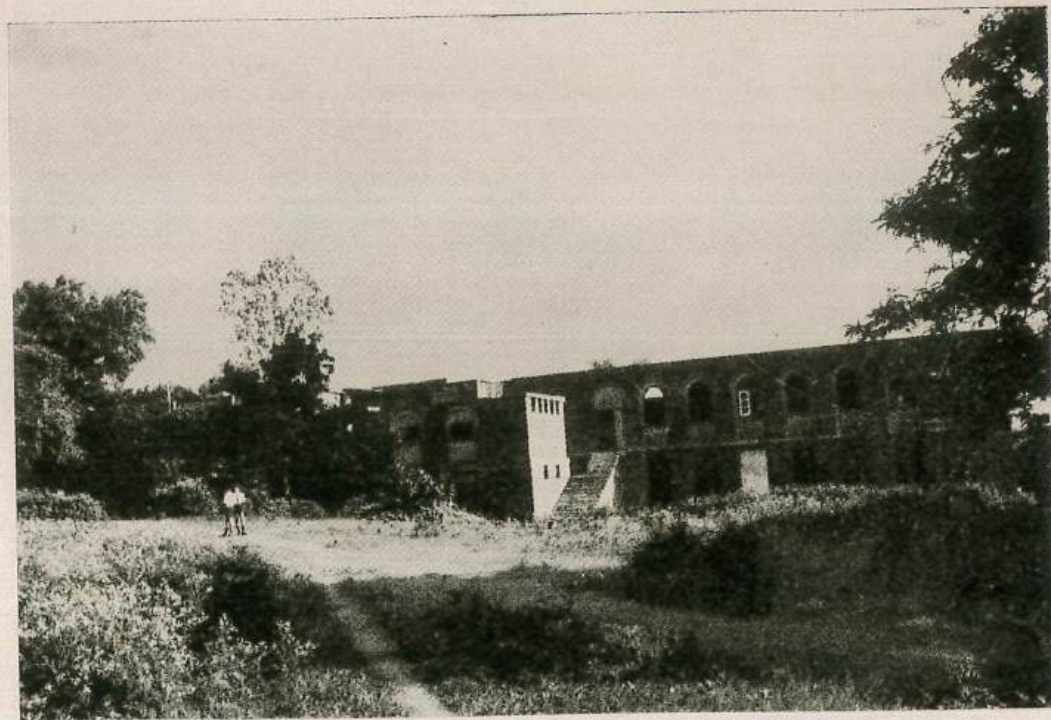
Incomplete block with the Laboratories.
