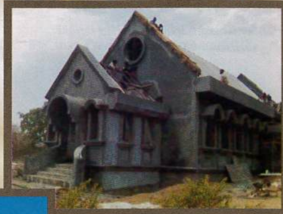
The Chapel construction work in progress.
