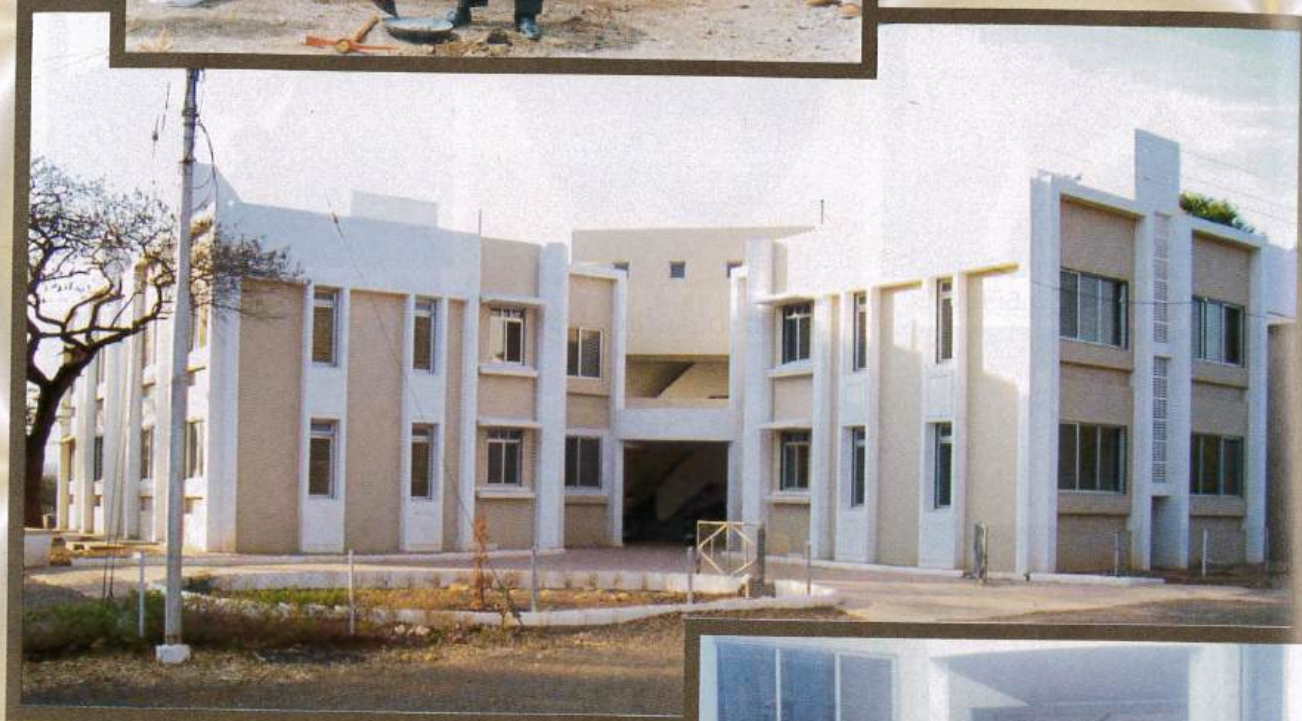
The completed new staff quarters.
